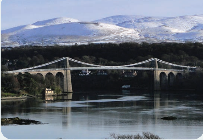
The Menai Suspension Bridge, UK, designed by Thomas Telford and completed in 1826, features large amounts of wrought iron. Courtesy of Bencherlite.
