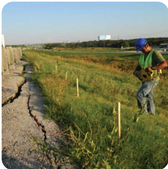
Sadik Khan, Sahadat Hossain's doctoral student, views a failing slope along U.S. Route 287.
