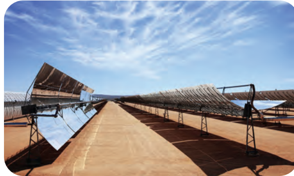
Solar power reflectors collect dust and sand, reducing their energy efficiency—a challenge ORNL researchers are tackling by developing a low-cost, anti-soiling coating.
