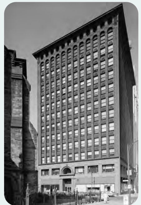
Architect and "father of skyscrapers" Louis Sullivan's Prudential Building, Buffalo, N.Y. Courtesy of Library of Congress/U.S. public domain.
