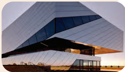
The unusual design of the Paläon with ALUCOBOND panels won the 2013 German Facade Award for rainscreen cladding.
