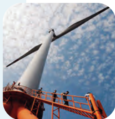
Two-bladed wind turbines, like this one in China, could lower the cost of wind power.
