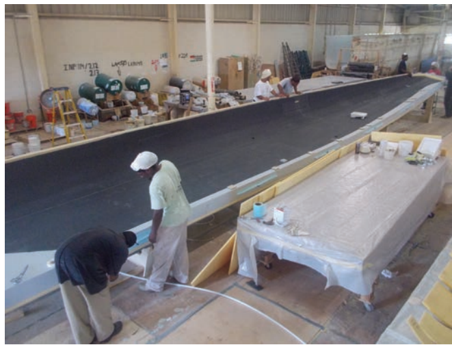
B53 under construction.
