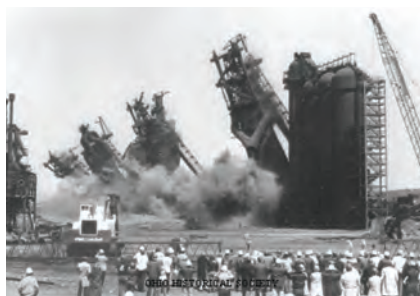
Demolition of three blast furnaces at the Ohio Works in Youngstown in 1984. Courtesy of urbanohio.com.
